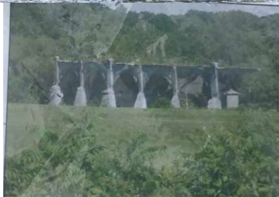
The six arches of the old Schoharie Aqueduct, a National Historic Landmark.
